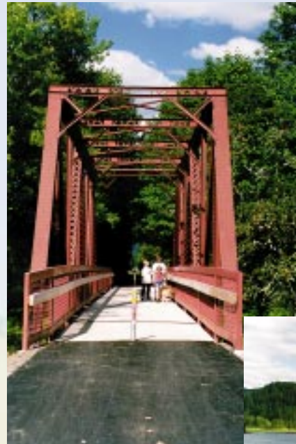
Mosby Creek Bridge
